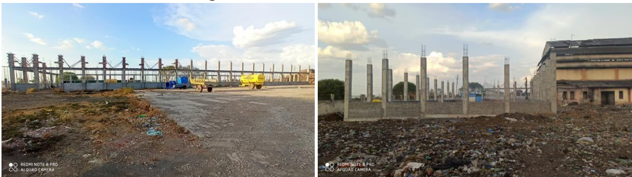
Figure 10: New shed for storage
