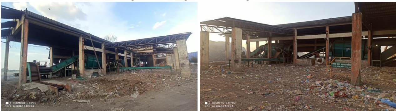
Figure 8: Existing machinery on site
