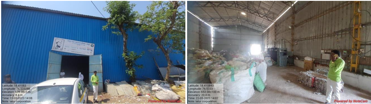
Figure 7: Existing MRF Processing shed
